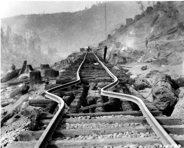
Image: "215533 Rails Buckled after Trestle Fire, Pe Ell, WA 1926 „ by Forest Service via Flickr https://www.flickr.com/photos/forestservicenw/21851483880/ Creative Commons Attribution 2.0 Generic (CC BY 2.0) https://creativecommons.org/licenses/by/2.0/
